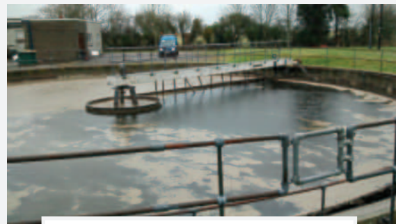
Figure 7. Secondary Clarifier Before Trial
