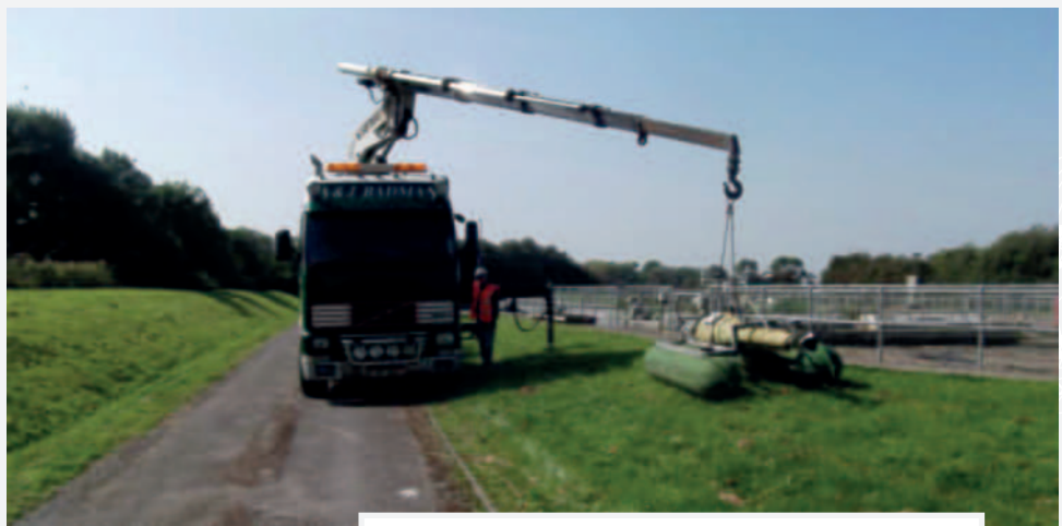
Figure 9. Aerator removed for maintenance and repair
